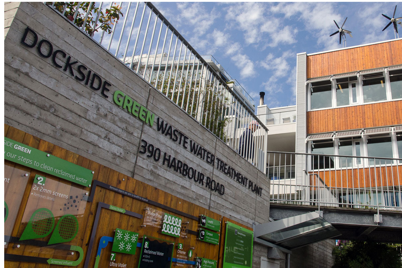
WASTE WATER TREATMENT FACILITY, DOCKSIDER GREEN
