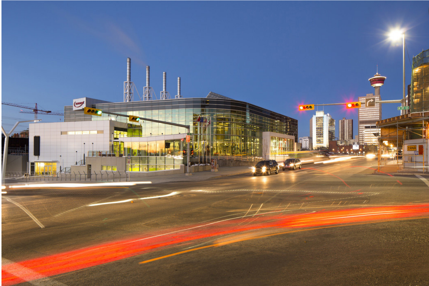
ENMAX DISTRICT ENERGY CENTRE, CALGARY
