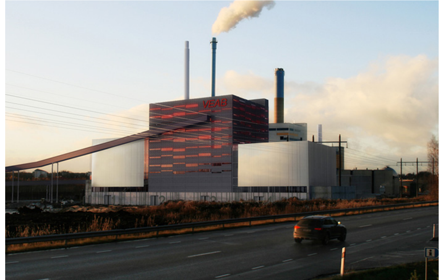
SANDVIK CHP STATION, SWEDEN
