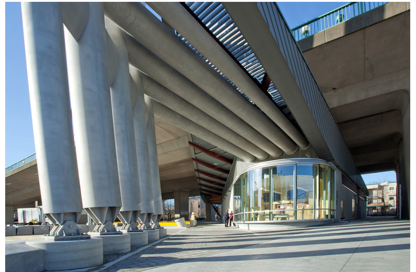
SOUTHEAST FALSE CREEK ENERGY CENTRE, VANCOUVER
