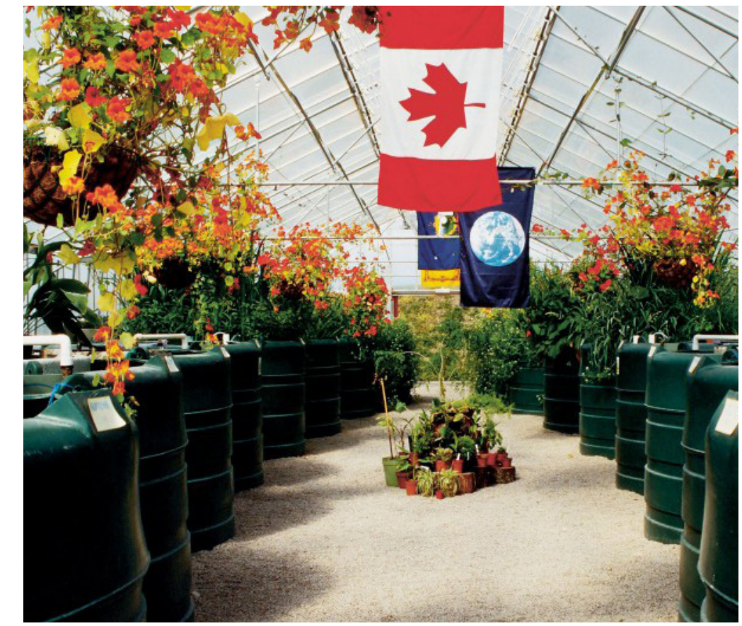
Image: Findhorn Living Machine in Ecovillage, Moray, Scotland Living machines use plants to naturally filter waste from water.
