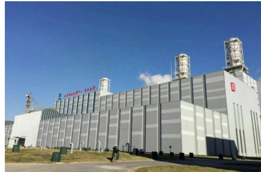
Combine heat and power (CHP), Peking City, China (source: https://www.powermag.com/optimizing-combined-heat-and-power-in-china/ )
