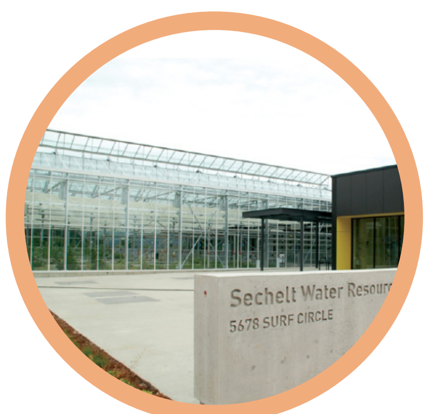
SECHULT WASTE WATER PLANT (VANCOUVER)
