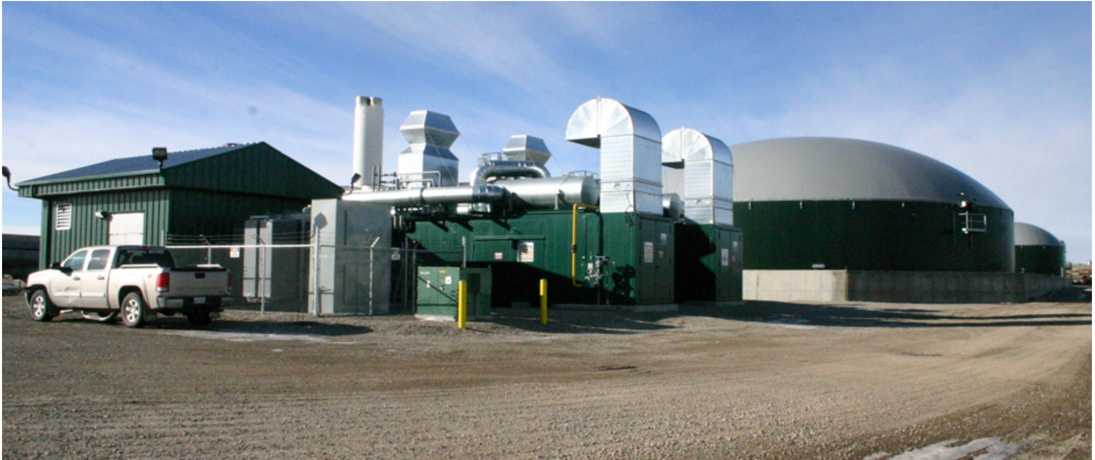
Biogas Plant, Lethbridge, Alberta
