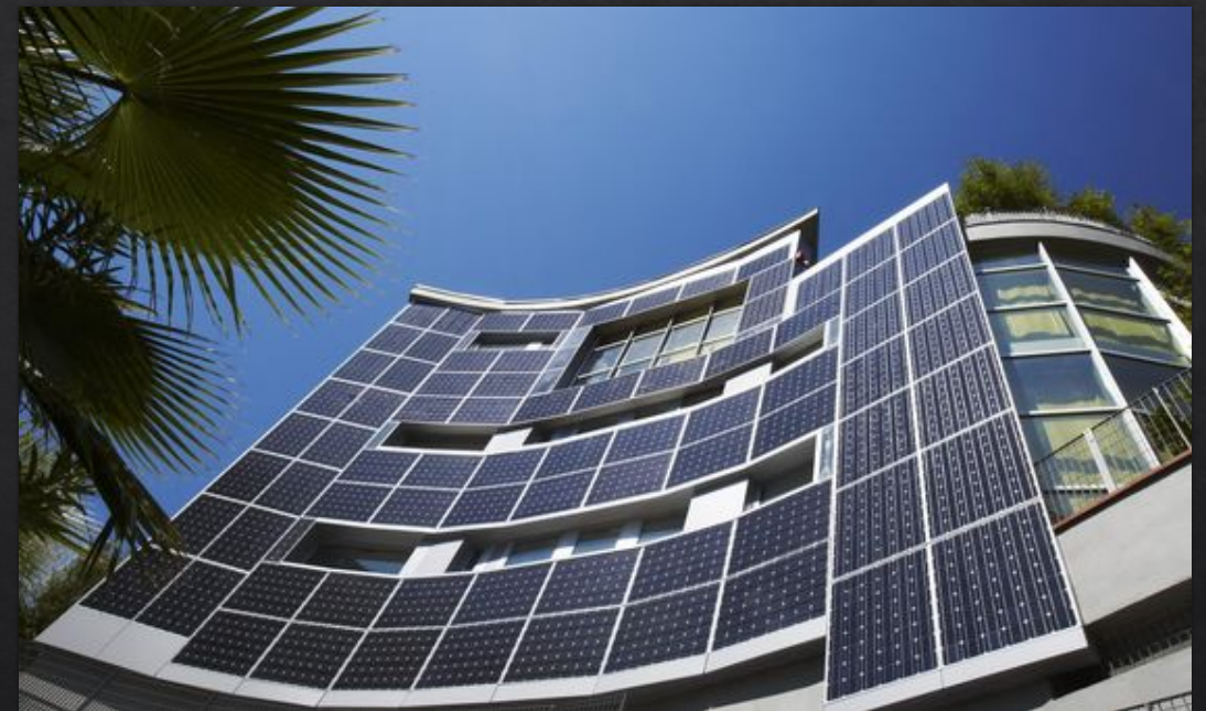
Building Façade Integration – 5% coverage
